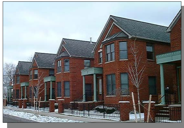
Example of multiple family housing
